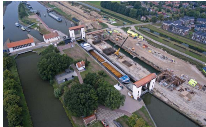
The lock in Eefde (Netherlands) was built in 1933 and is now extended by another lock chamber.
