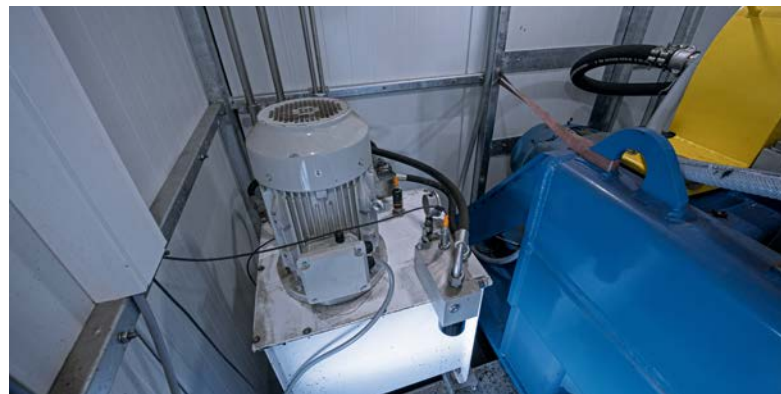
The electrically driven hydraulic unit for the screw conveyor in the centrifuge.
