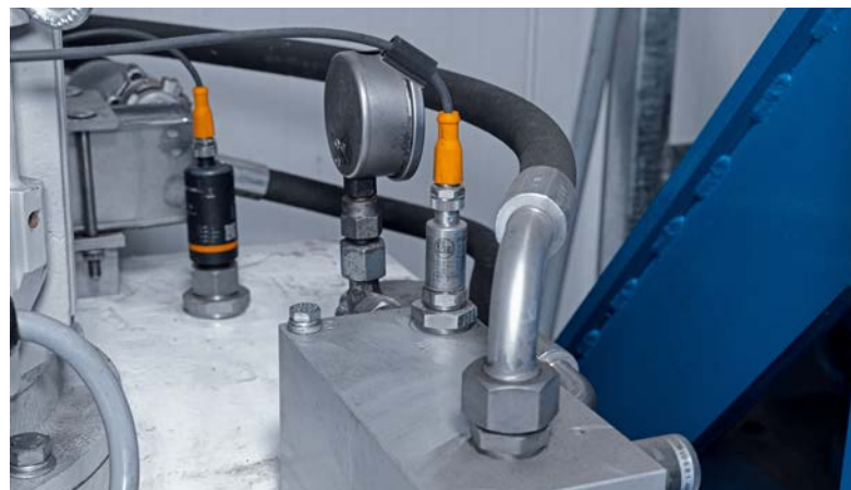
Monitoring of the hydraulic aggregate with regard to pressure, oil level and temperature.
