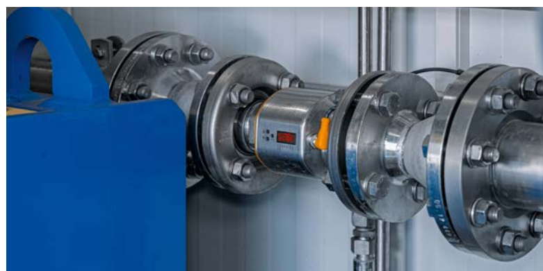
Central measured value: A magnetic-inductive flow sensor monitors the amount of sewage sludge entering the centrifuge.
