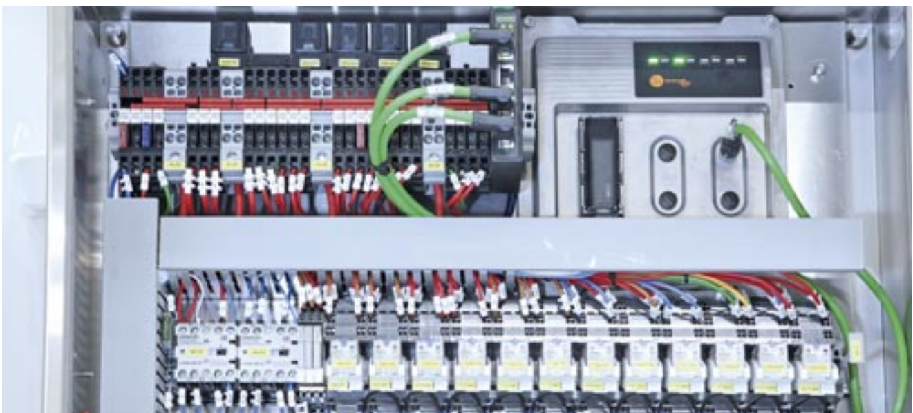
The core element at the top right of the control cabinet: the powerful ecomatController CR711S with two integrated PLCs (1x standard, 1x safety).
