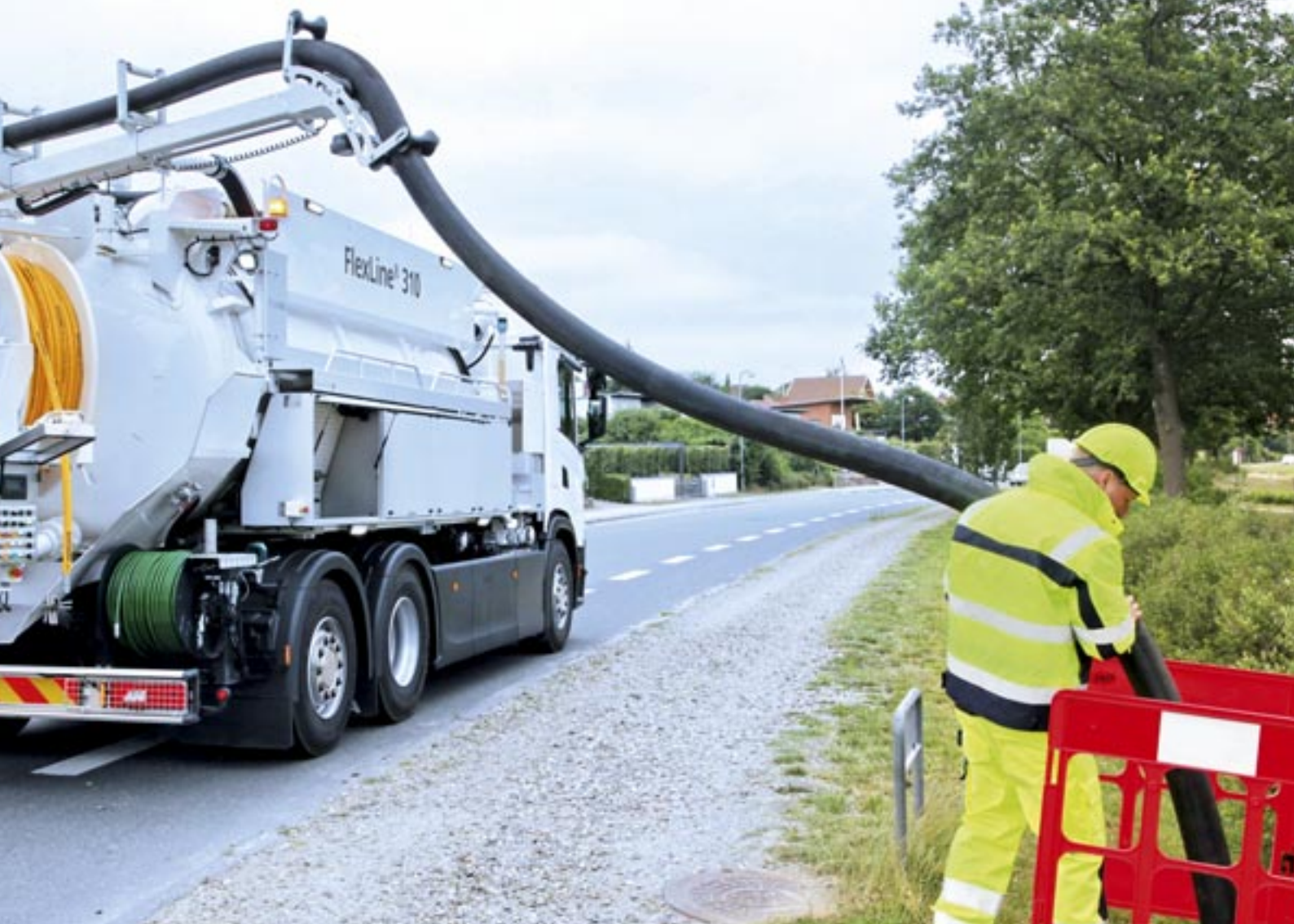
A sewer cleaning vehicle with the uncoiled jetting and suction pump for sewer cleaning.
