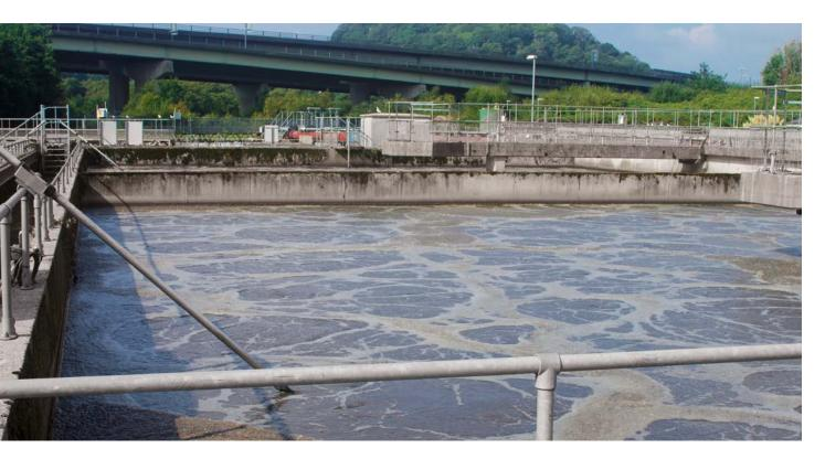
Air is pumped into the aeration basin via powerful blowers – up to 390 cubic meters per minute at Marsh Mills.
