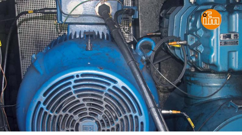
Vibration sensors on the motors of the blowers detect incipient defects well before major damage occurs.
