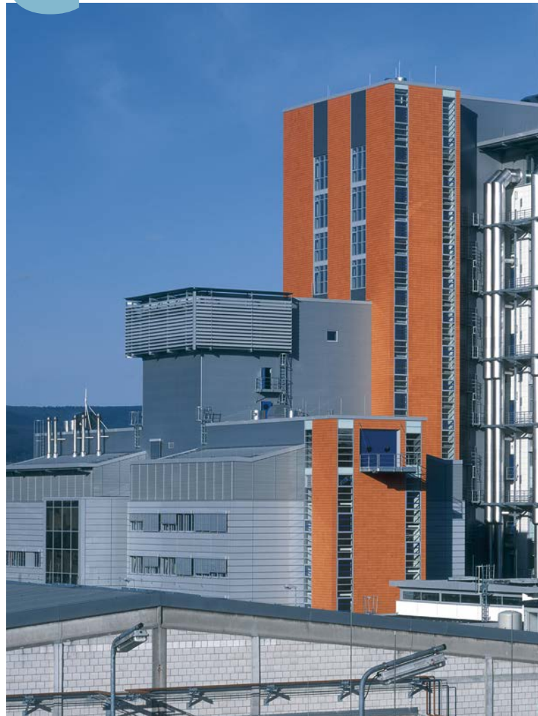
The pharmaceutical company Boehringer Ingelheim relies on vibration diagnostics from ifm for condition-based maintenance in its cleanroom ventilation systems.
