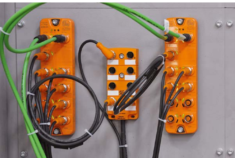
The information from the sensors is bundled in IO-Link masters and forwarded from there via an IoT connection (green cable) for IT-based evaluation.
