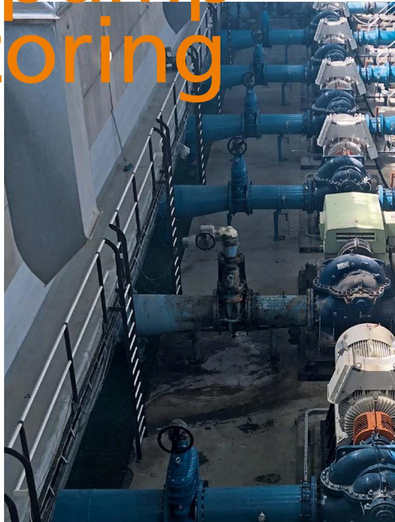
*The high-lift pump station of Midvaal Water. The five newer motor-pump sets (grey motor housing) were equipped with IO-Link sensors and condition monitoring solutions.*
