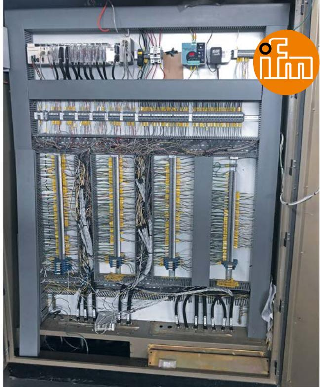
Before using IO-Link, two of these cabinets with analogue cards were needed to record the values of the sensors.
