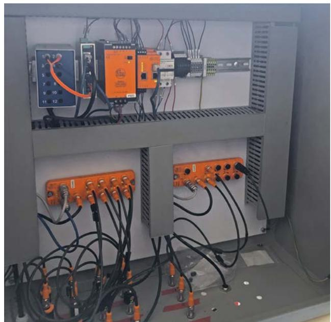
With IO-Link, fewer cables and less space are required. Midvaal Water was able to reduce installation time by 80 percent.
